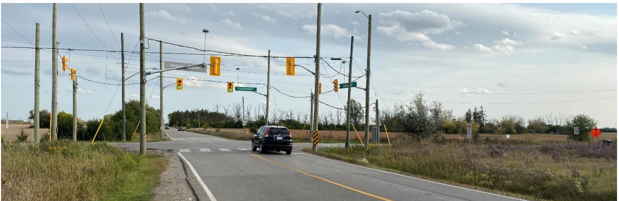
Image 9: Coleraine Drive and Countryside Drive Intersection – Looking South
