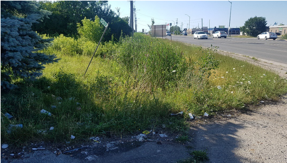
Image 5: View of disturbances associated with the asphalt roadway and driveway, paved shoulder, culvert, and wet ditching.
