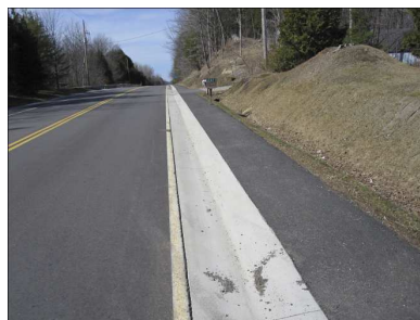
Examples of rural road reconstruction/rehabilitation within the Region of Peel,
