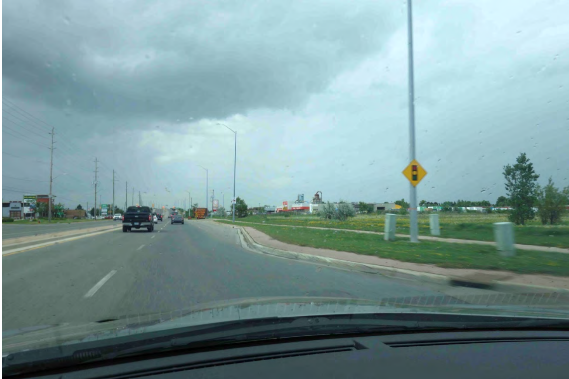
HIGHWAY 50 TRAVELLING NORTH FROM McEWAN DRIVE
