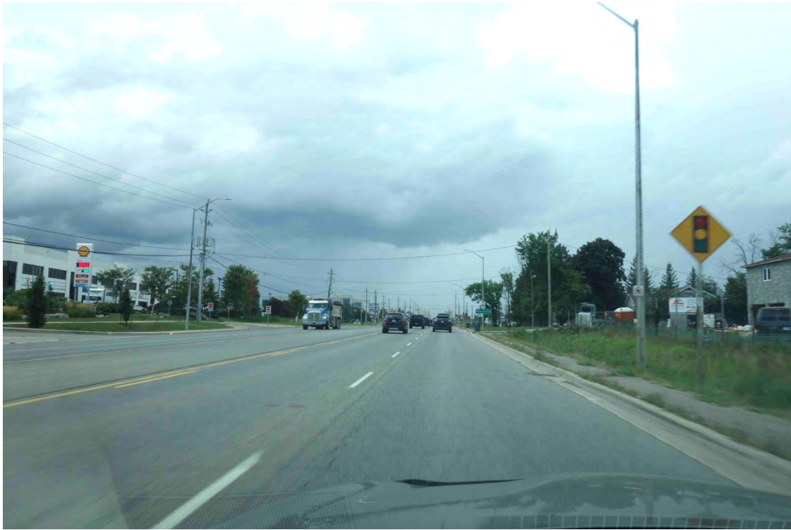
HIGHWAY 50 TRAVELLING NORTH FROM MAYFIELD ROAD
