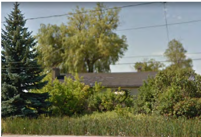
12532 HIGHWAY 50 – early 20 th century dwelling
