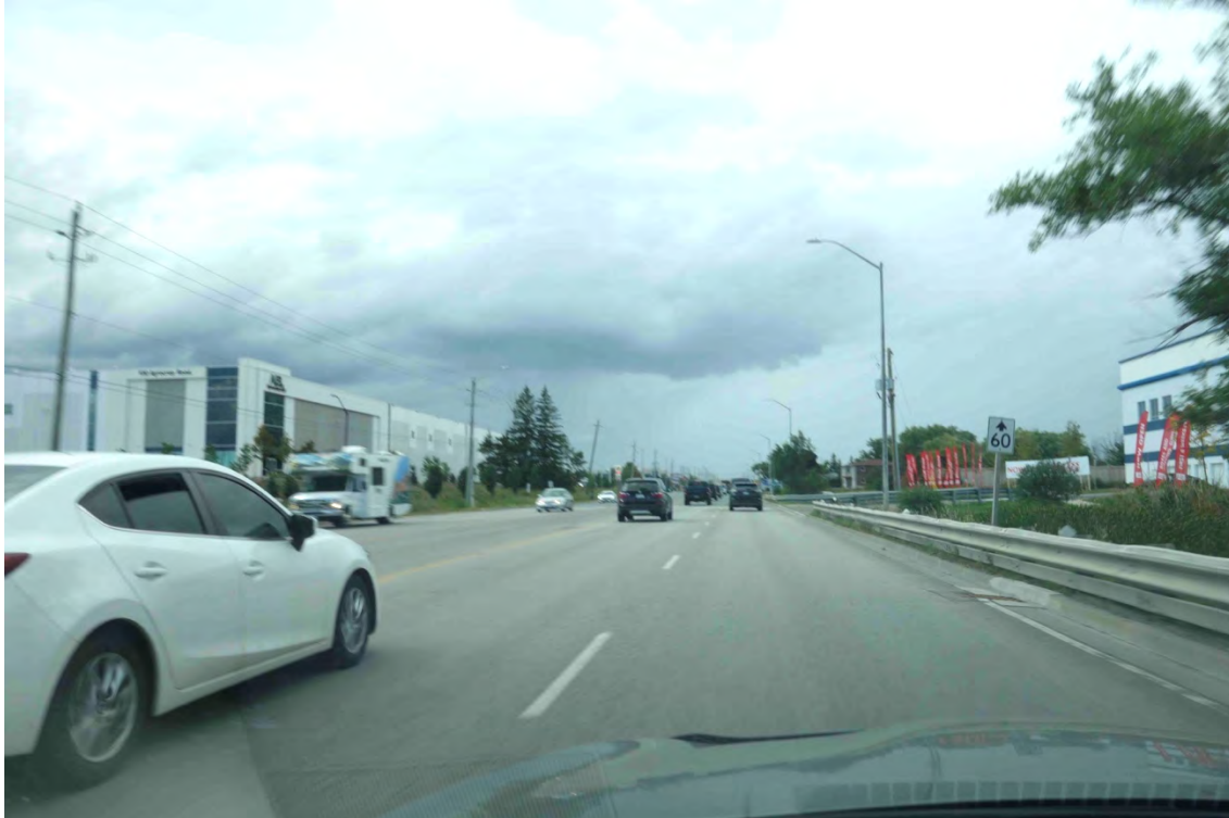
HIGHWAY 50 TRAVELLING NORTH FROM MAYFIELD ROAD
