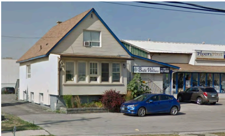
12388 HIGHWAY 50 – early 20 th century residence converted for commercial use
