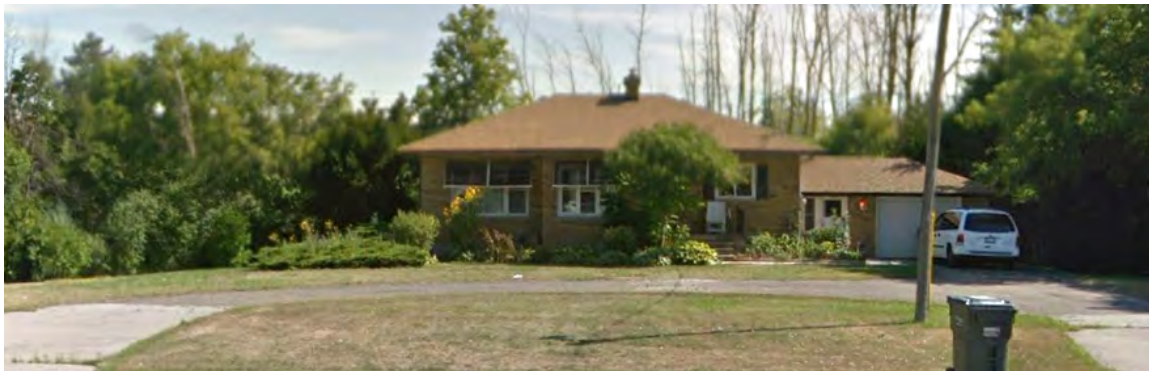
12207 HIGHWAY 50 – mid-20 th century dwelling
