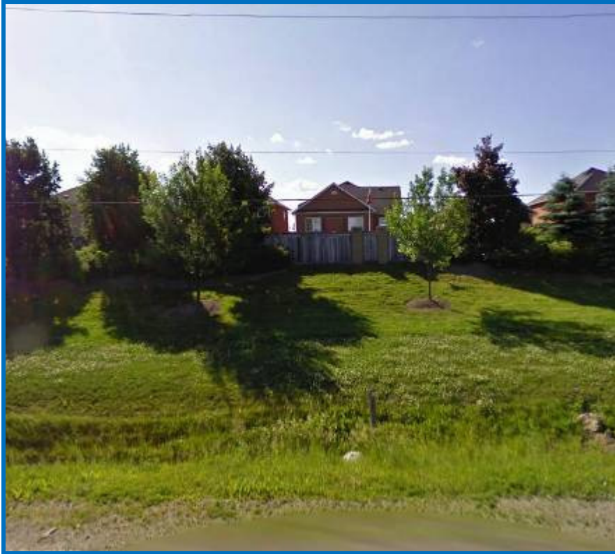
Figure 3 Wooden fence constructed on an elevated slope, viewed from Mayfield Road.
