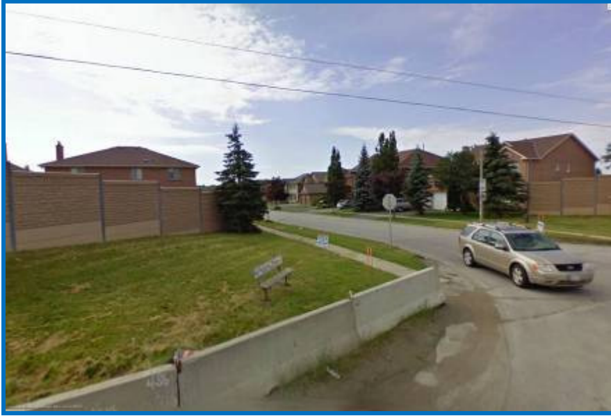
Figure 5 Noise Barrier along south side of Mayfield Road at Stonegate Drive.
