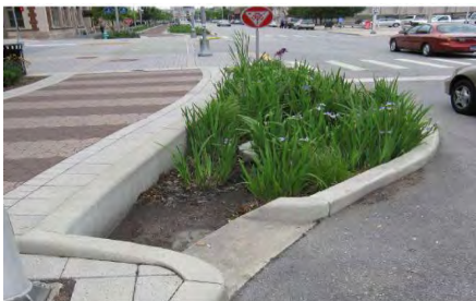
Example 1 of Stormwater Management
