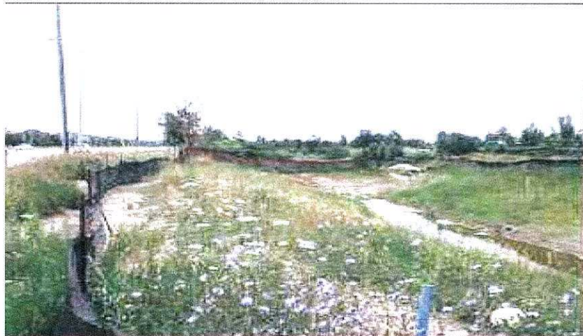
Looking south on west side of Dixie Road at altered watercourse
