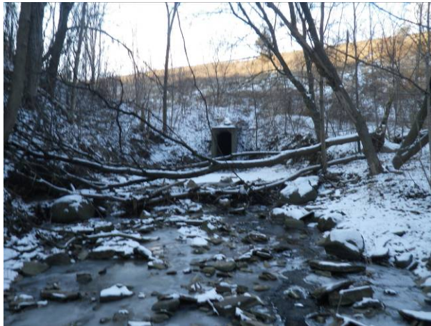
View facing upstream at the Bovaird Drive culvert outlet. It is evident that the culvert is undersized in relation to the existing watercourse. Scour along bed and banks of channel have resulted.
