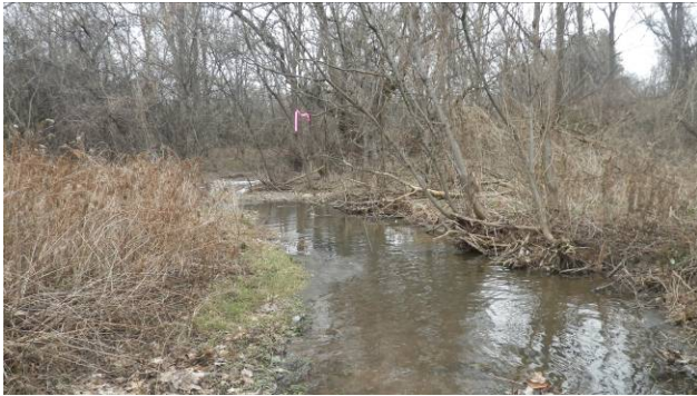
XS 9: View facing upstream. Slopes are gradual, some leaning trees can be observed on the bank (left bank).
