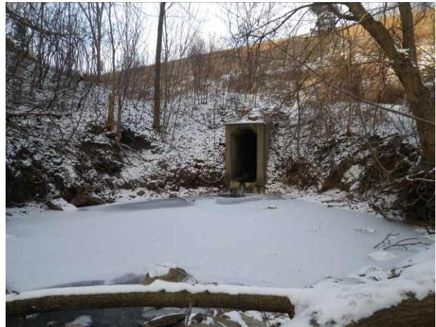
View facing upstream at the Bovaird Drive culvert outlet. It is evident that the culvert is undersized in relation to the existing watercourse. Scour along bed and banks of channel have resulted.
