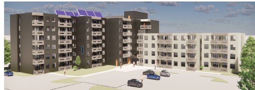
Hillside Place, Mississauga - Full envelope restoration to set up building for future low carbon retrofits by increasing air tightness of the building envelope
