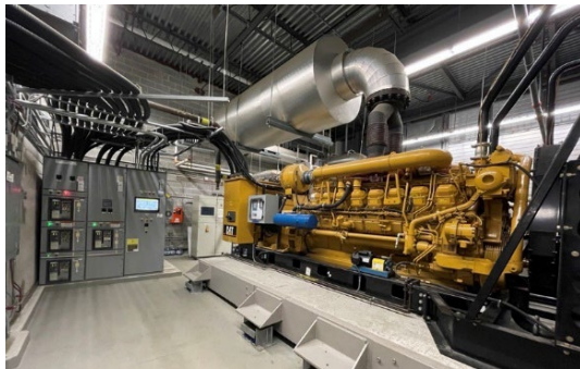
Technical breaker maintenance
